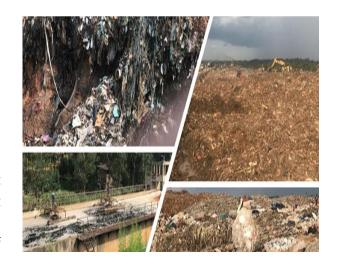
sanitary engineered landfill and has now reached its maximum capacity with the height of the landfill, steep slopes and the lack of compaction giving rise to stability concerns.
